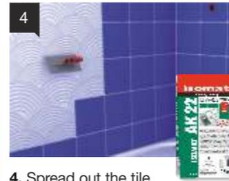
4. Spread out the tile adhesive **ISOMAT AK 22** and fix the tiles.
