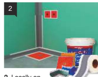
2. Locally on pipe entries, floor drains etc., apply one layer of **ISOMAT SL 17** and, while still fresh, embed the joint sealing tape or sealing collars.
