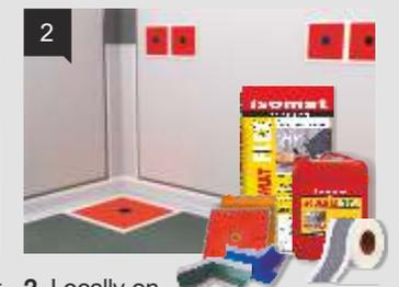
2. Locally on pipe entries, floor drains etc., apply one layer of **AQUAMAT-FLEX** and, while still fresh, embed the joint sealing tape or sealing collars.
