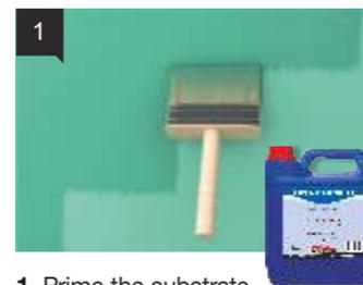
1. Prime the substrate (cement mortar, gypsum board, plaster, etc.) with the acrylic primer **UNI-PRIMER**.
