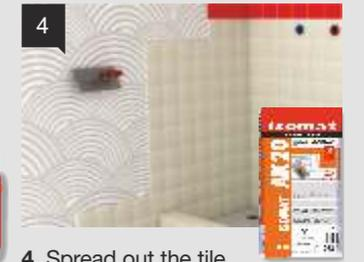
4. Spread out the tile adhesive **ISOMAT AK 20** and fix the tiles.
