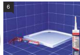
6. Finally, seal the intersections with **DOMOSIL-MICRO**.
